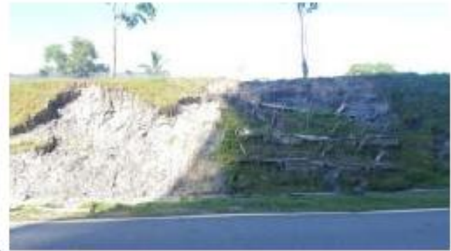
Photo Description: Slope 1 – Height : 4m. Width : 19.1m.
